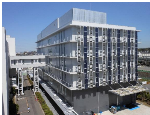
Building No.502 at the Yokohama Plant
