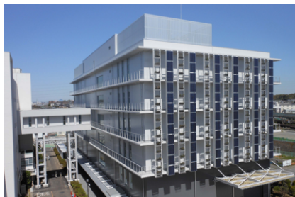
Solar panels on the wall of a building of Nikon Yokohama Plant
