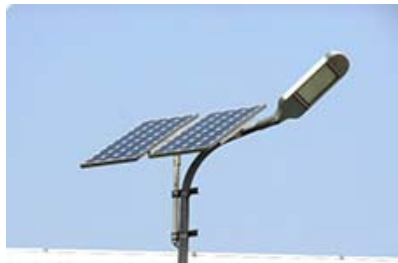
LED outdoor lighting with solar panel at Nikon Imaging (China) Co., Ltd.
